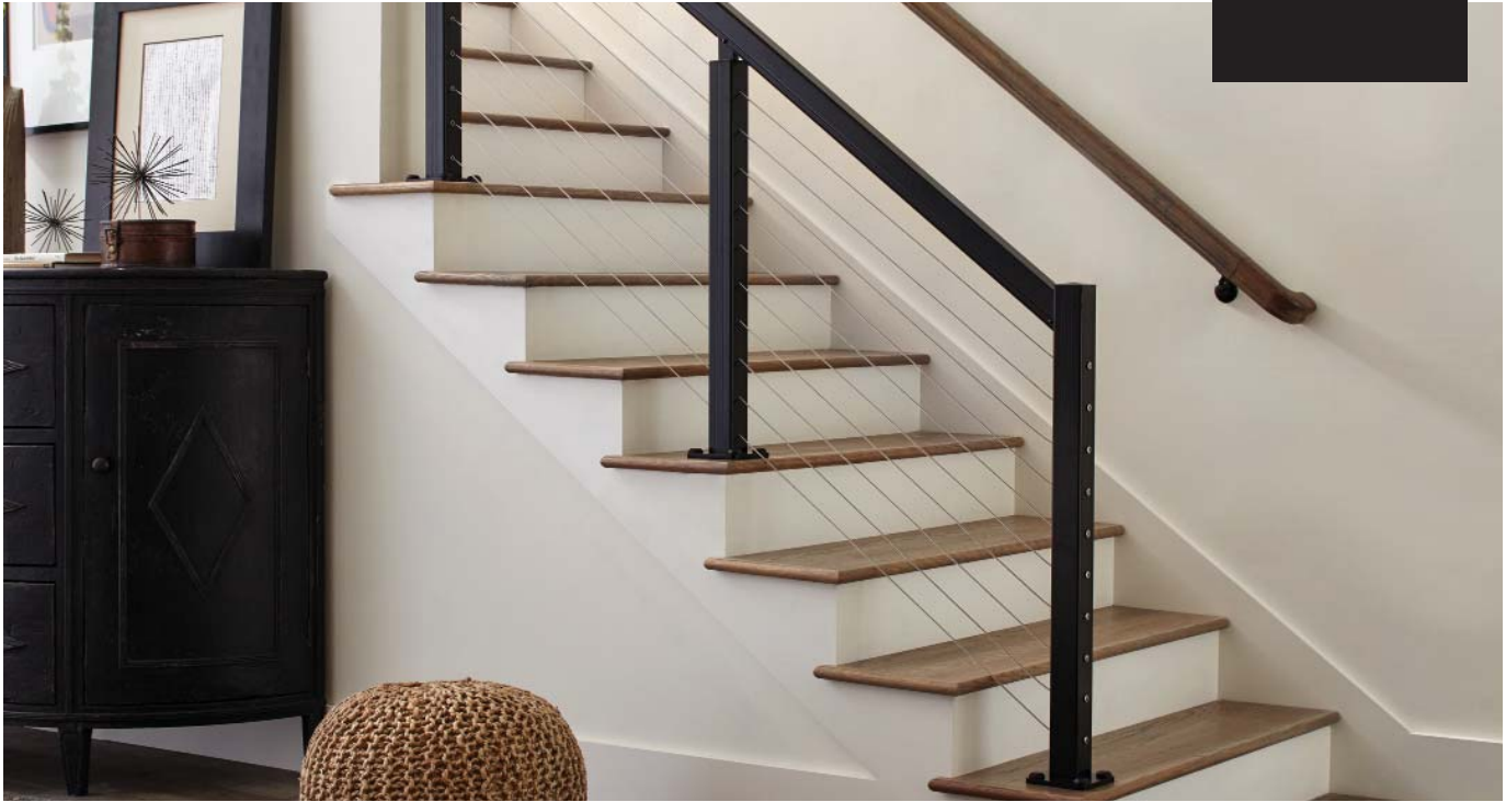
Pictured using intermediate post fitting (Item #0412) and post cap (Item #0410).
