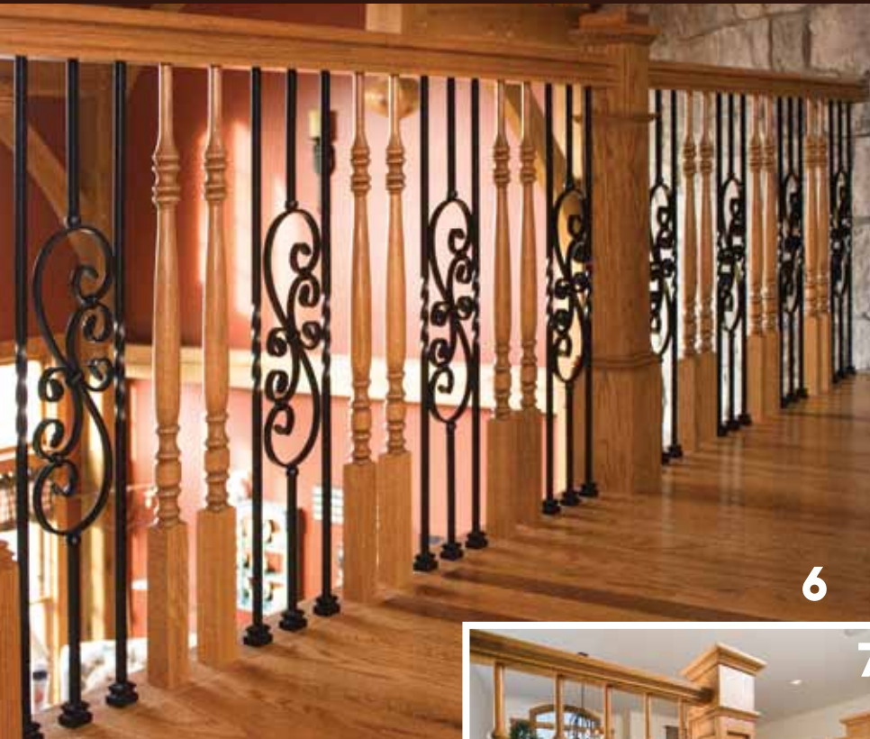
6 LJ-5300 Wood Balusters, LI-1TW44 & LI-50144 Iron Balusters, LJ-4091 Box Newel and 6519 Handrail
